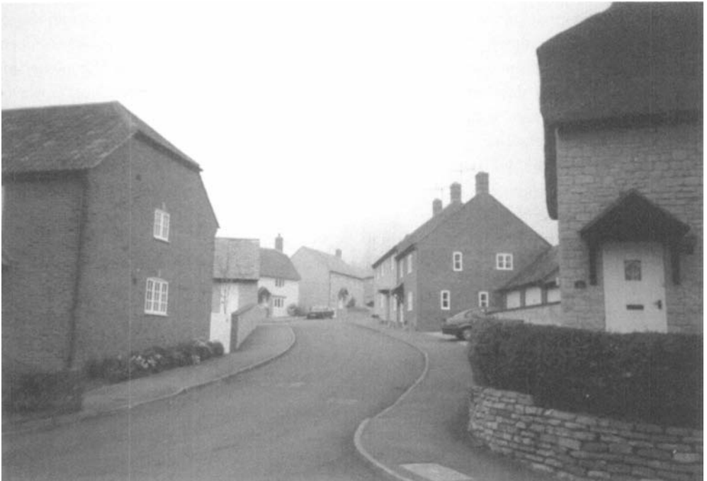
Figure 8.2 New housing in the village of Burton Bradstock, Dorset, built in the local vernacular using reconstituted stone
