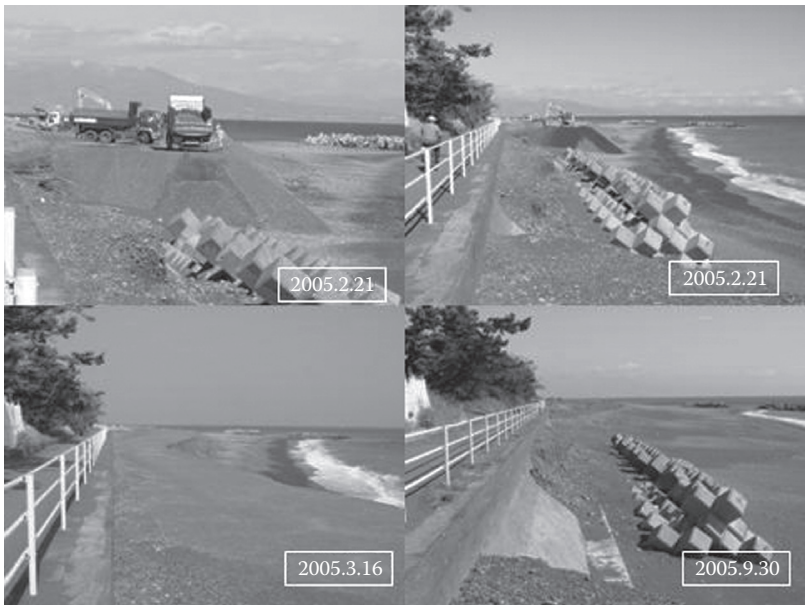
FIGURE 8.21 Countermeasure for coastal erosion by dumping and the action of erosion.
